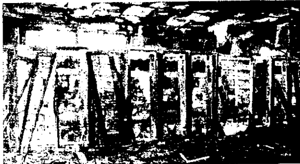
The control room of Sharavathi hydroelectric plant at Jog Falls in Shivamogga district which was damaged in the fire on Thursday. (The Hindu)
